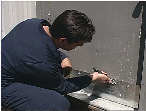
**Excluding rodents from layer houses means making sure doors close all the way and patching any holes in the exterior of the building with rodent-proof materials. Photo courtesy of Motomco**
